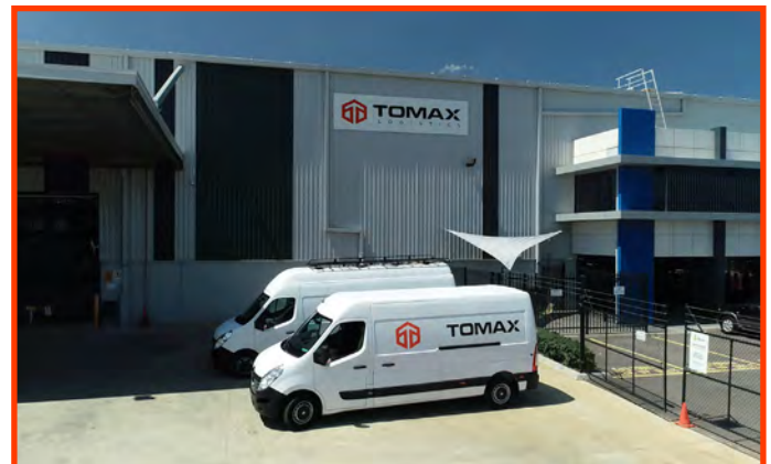
Tomax Dandenong South Warehouse
